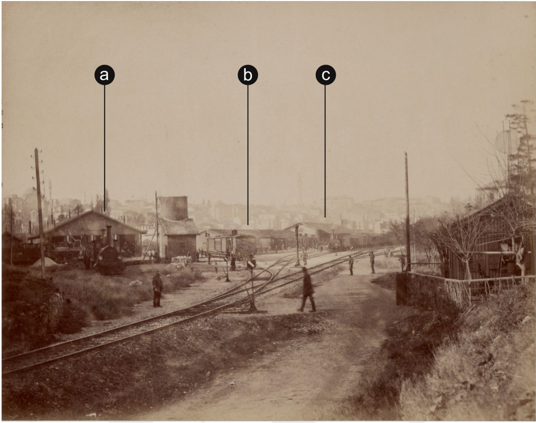
Figure 11. Commercial and technical buildings in the railway compound. Legend: (a) Locomotive shed, (b) provisional storage, (c) merchandise shed and customhouse. Source: Istanbul University Rare Materials Collection, 91545/008.
