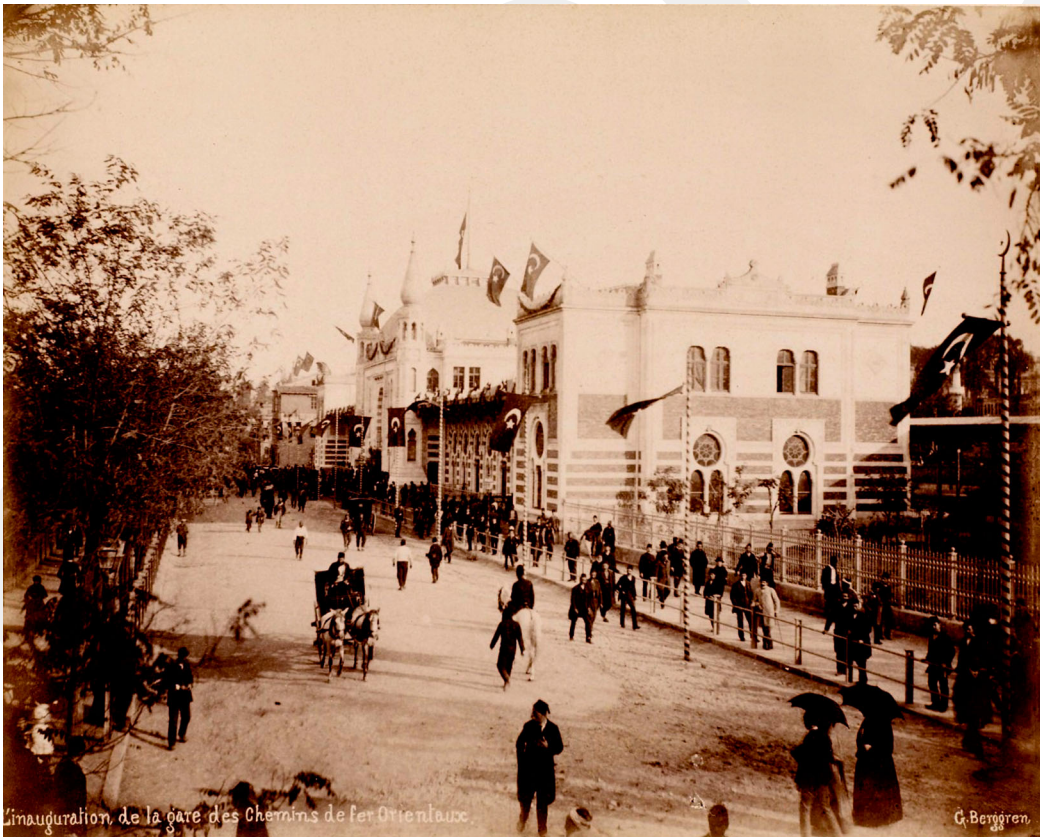
Figure 14. The inauguration of passenger station, 1890. Source: Author's collection.
