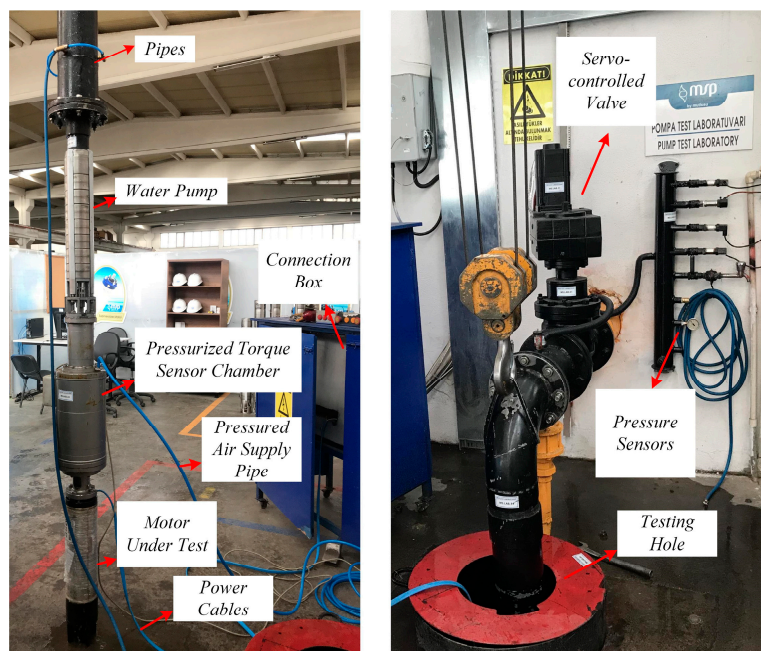
Figure 8. Motor under test, torque sensor, pump assembly, servo-controlled valve, pressure sensor, flowmeter, and auxiliary tank arrangement.
