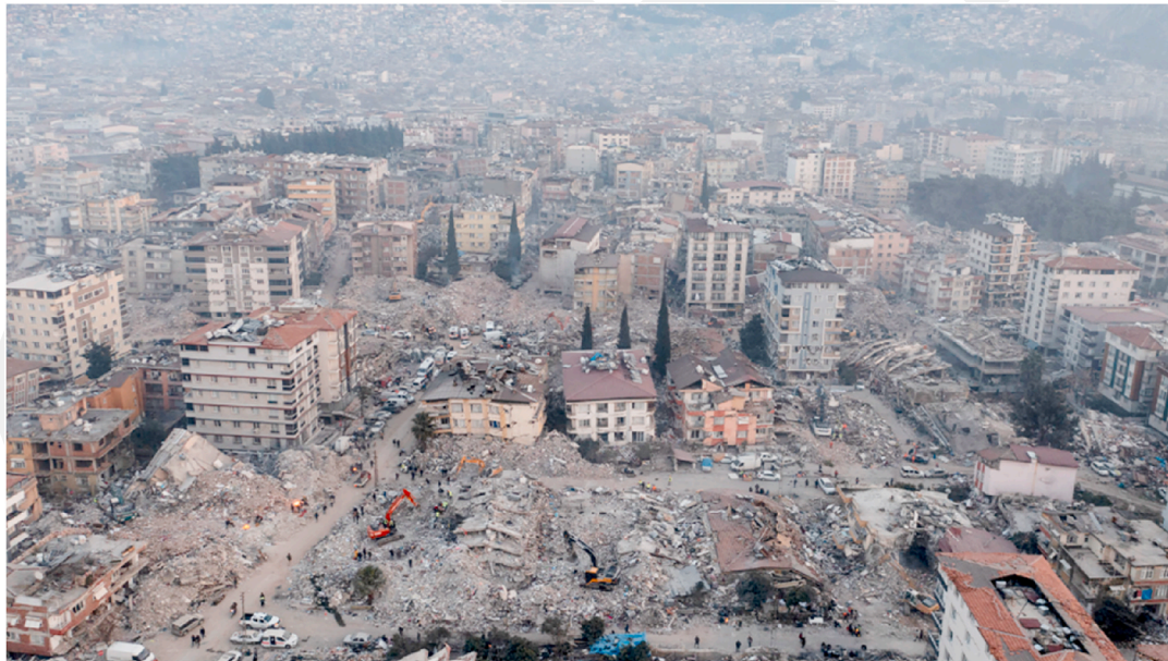
Fig. 4. Destruction in Kahramanmaraş due to earthquake on 6th February of 2023.
