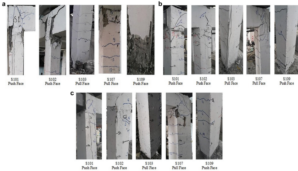
Figure 10. (a) Damage appeared in some columns of the reference frame at the end of the test. (b) Damage appeared in some columns of the strengthened damaged frame at the end of the test. (c) Damage appeared in some columns of the strengthened undamaged frame at the end of the test.
