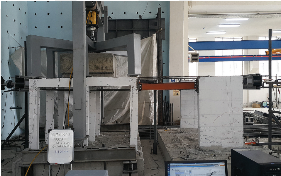
Figure 8. The appearance of the strengthened damaged frame at the end of the third test.
