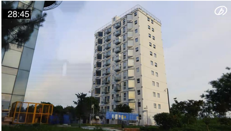
Figure 4.4.8 Ten floor stainless-steel modular building in 28 hours ( Ten-Storey Stainless-Steel Apartment Block Built in 28 Hours , n.d.)
