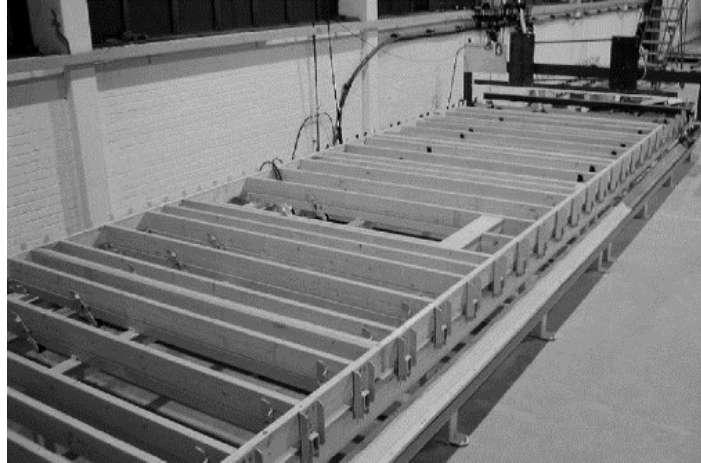
Figure 3.3.2 Manufacturing a timber floor (Lawson et al., 2014)
