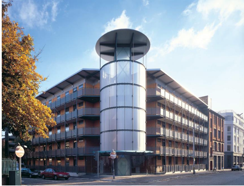
Figure 4.3.2 Murray Grove building in Hackney, London (Pickard, 1999)
