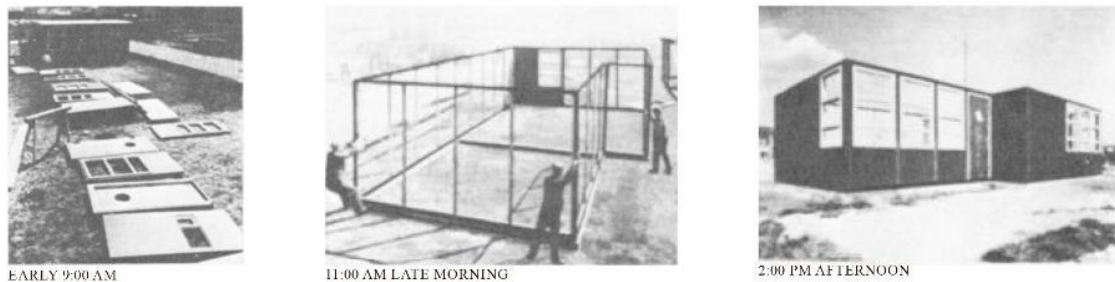
Figure 2.3.7 Copper house erection speed process, Berlin exhibition 1932 (Gropius & Wachsmann, 2021).
