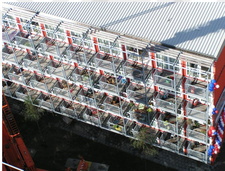
Figure 3.3.8 Keetwonen Amsterdam, reused shipping containers modules (P-34, Tables 4.1.1 & 4.1.2)
