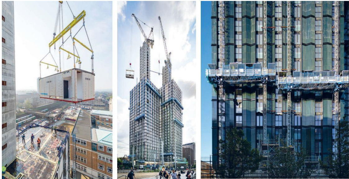
Figure 4.3.9 The construction process of Ten Degrees, craning, installation of modules, and façade works (Bayliss & Rory, 2020)
