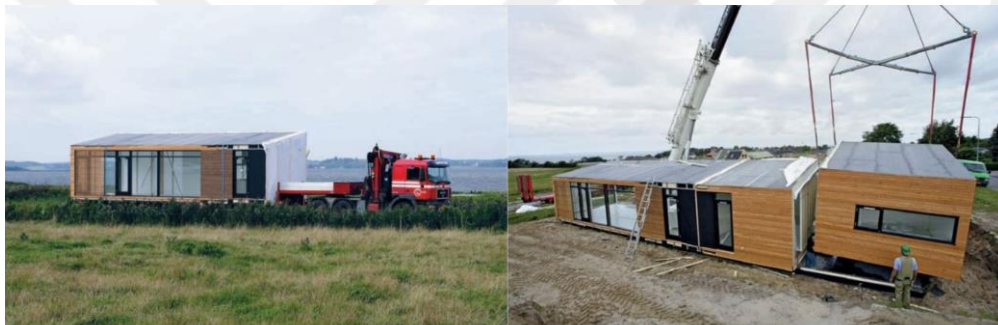
Figure 4.3.15 Transportation and installation of ONV house modules (Staib et al., 2008)
