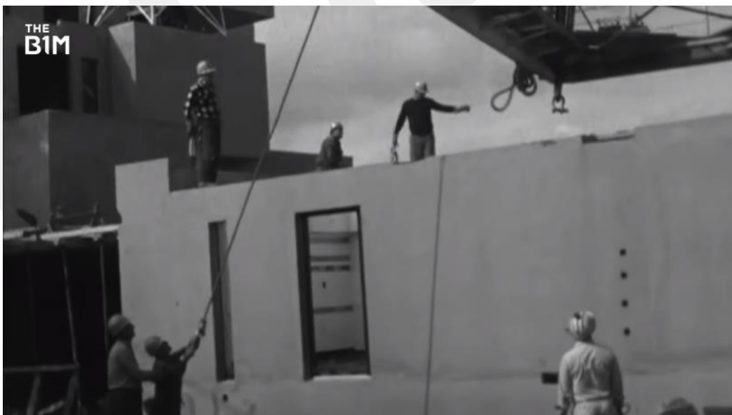
Figure 4.2.6 Workers during the construction of Habitat 67 (B1M, 2023)
