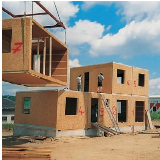
Figure 3.3.6 Timber module assembly process (Staib et al., 2008)
