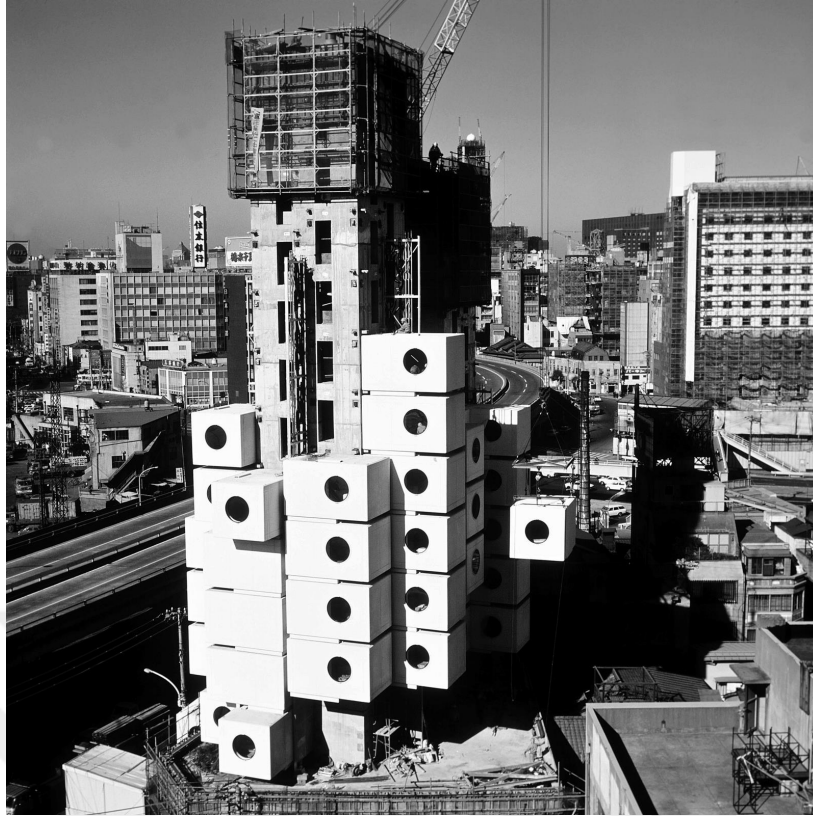
Figure 4.4.5 Nakagin Capsule Tower construction process (Lin, 2011)
