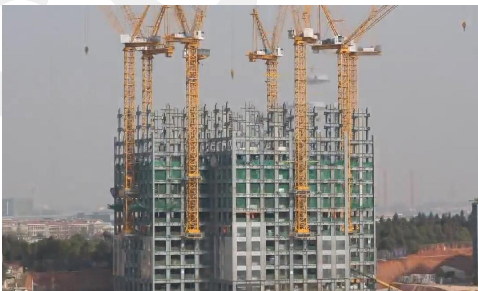
Figure 4.4.7 The 57 floor Mini Sky City erected in 19 days (The Mini Sky City, n.d.)
