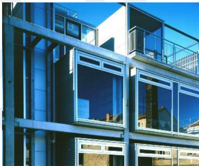
Figure 3.3.7 Modular housing project, Germany 1997, Steel room modules (P-10, Tables 4.1.1 & 4.1.2)
