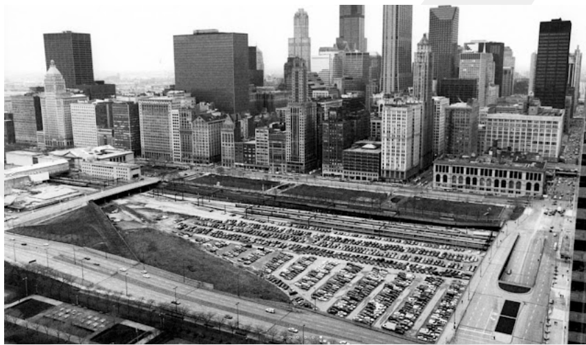
Figure 4.2. Illinois Central train yard Before High Line Construction
