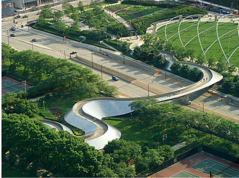
Figure 4.11 BP Pedestrian Bridge
