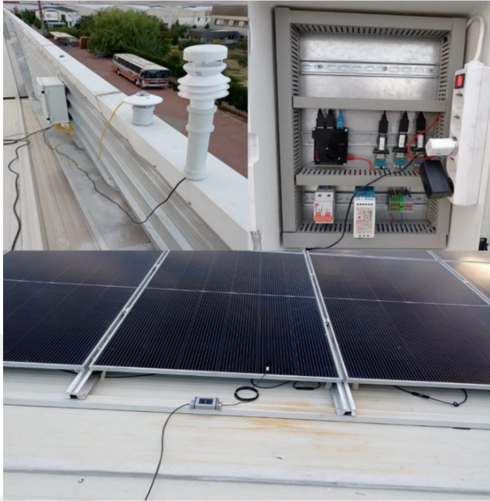
Figure 4.1 Sensors and Fisheye Camera Installation
