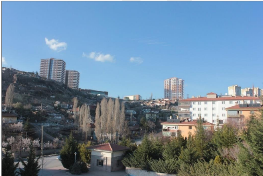
Figure 3 Partly demolished gecekondus and newly constructed apartments next to each other. Sinan Akyuz, 2016
