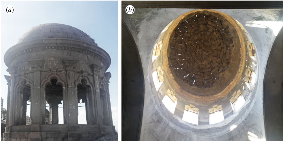
Figure 21. Oval dome of a run-down Orthodox church in Germin (Kayseri, Turkey). (a) External and (b) internal views. (Online version in colour.)
