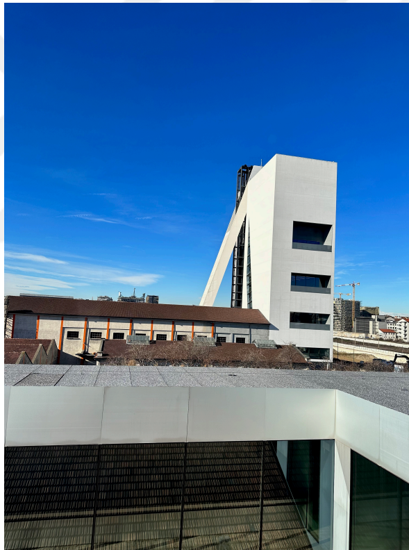
Figure 4.17 View of Fondazione Prada Torre Building from Haunted House, 24 th February 2023
