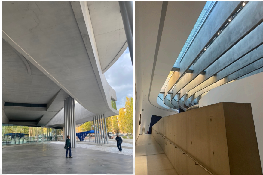
Figure 4.27 MAXXI Courtyard (left), MAXXI Interior (right), 7 th December 2022
