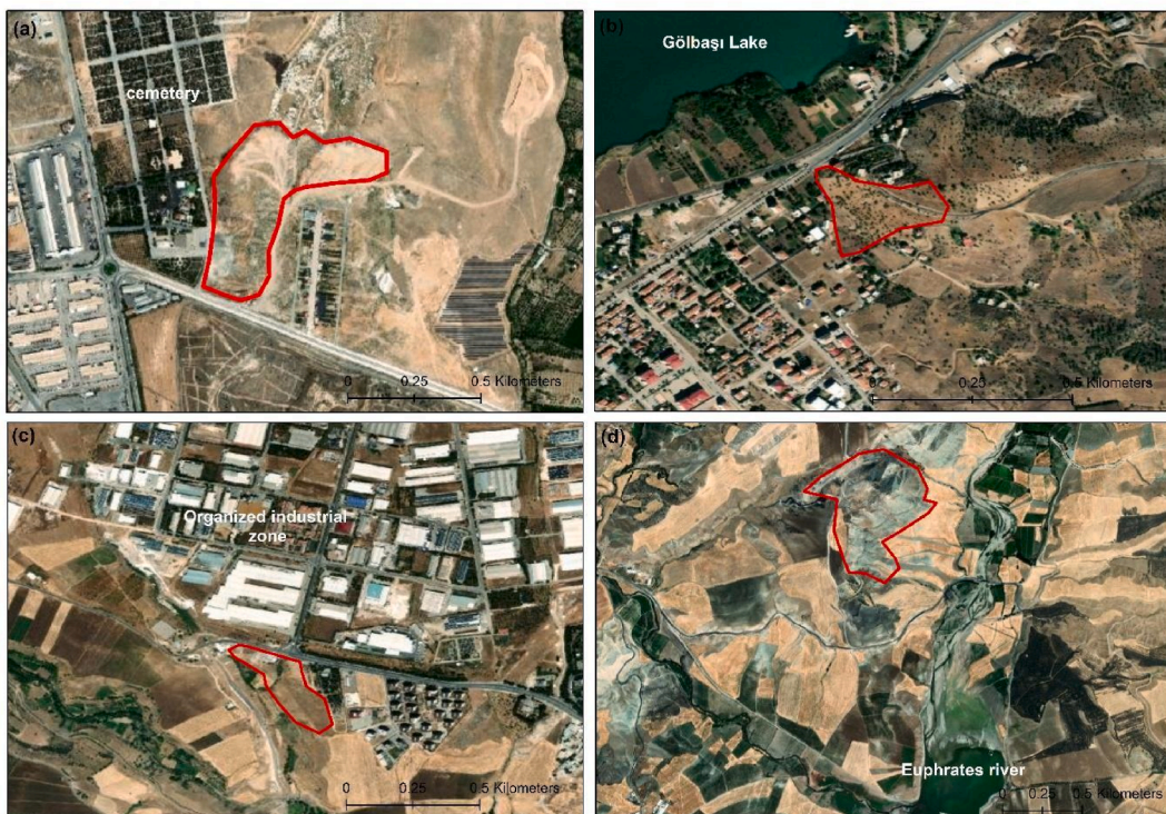
Fig. 3. Temporary disaster waste sites in (a) Malatya, (b) Gölbaşı, (c) Adıyaman near the organized industrial zone, and (d) Adıyaman on the old waste dump site.
