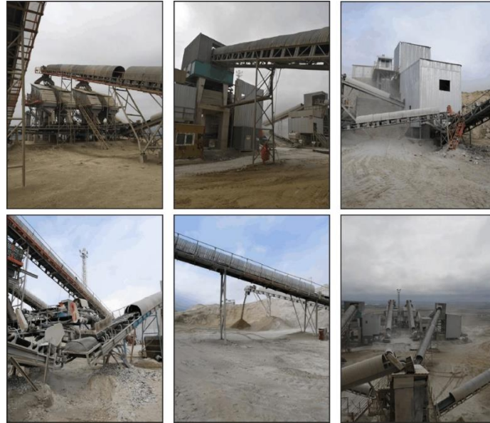
Figure 2. Typical inclined belt conveyors considered in this study.
