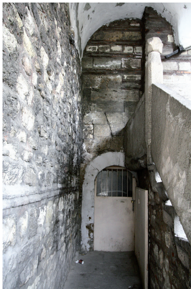
Figure 25. Relationship Between the Staircase and the Arched Door, 2012.
