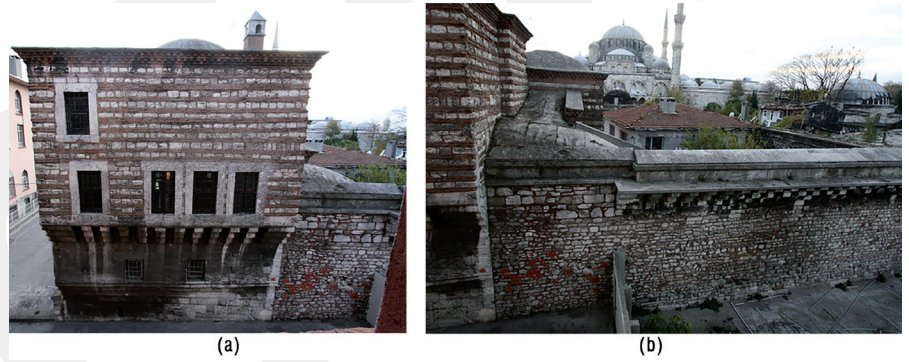
Figure 19. (a) Northeast Façade, (b) Garden Wall and Load-Bearer Stone Projections, 2012.
