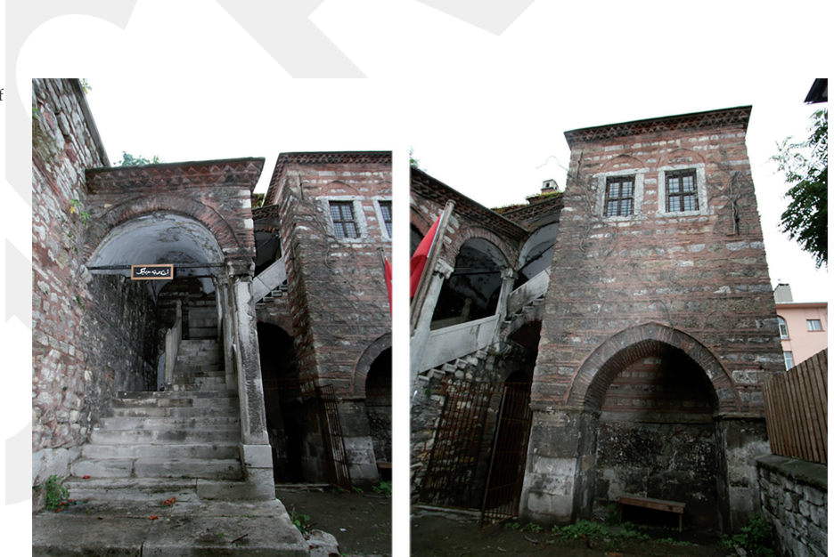
Figure 11. Samples of Wall Masonry Types of Şehit Ali Paşa Library, 2015.
